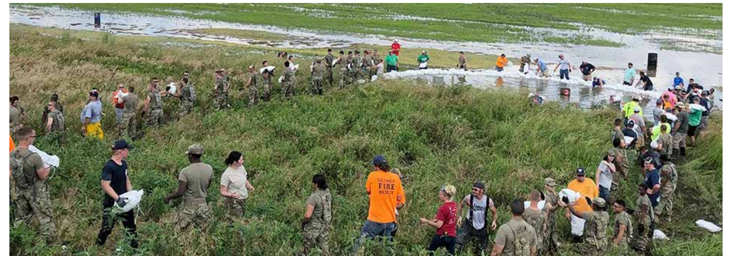
Below: The community works to stabilize the sand boil, 2019
